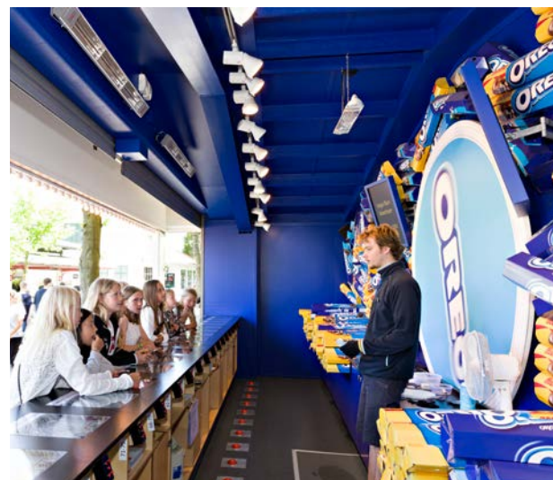
Radiant heaters are the perfect outdoor solution as they heat people and objects directly, not the surrounding air.
